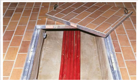
Multi-part cover for cable duct
